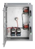
Pump control panel, Duplex controller NEMA size 0 Solid-state overload relay, OLR amp range 3-12A, 120 VAC coil, Fusible disconnect HOA Sel Sw. and Start P.B., Enclosure NEMA type 3/3R,12 Weather proof outdoor use
